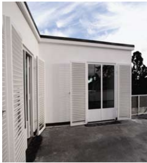
On the left: The house's western facade, with the steel stairway leading up to the roof terrace.
